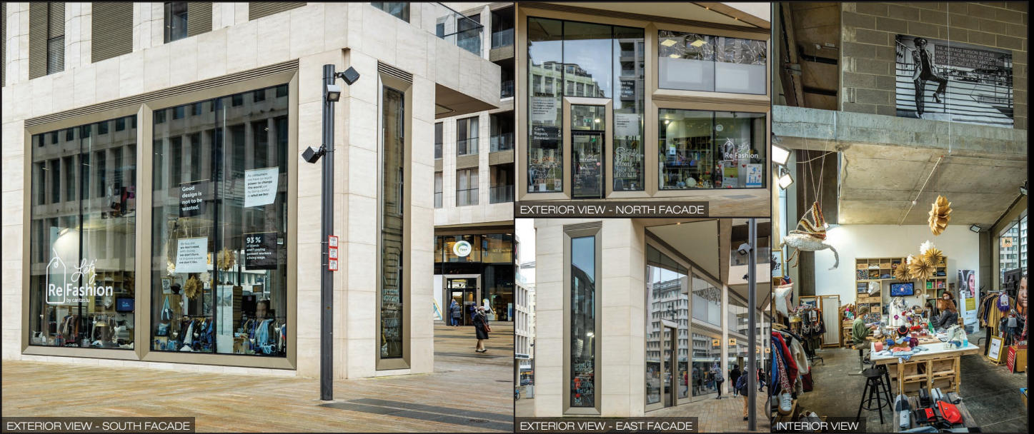
EXTERIOR VIEW - SOUTH FACADE
