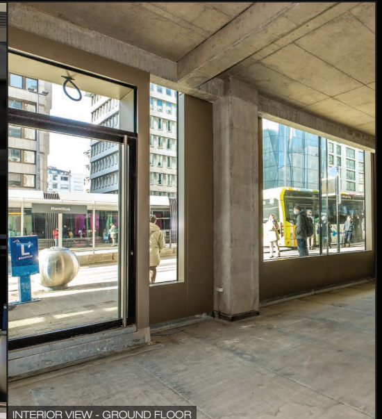
INTERIOR VIEW - GROUND FLOOR
