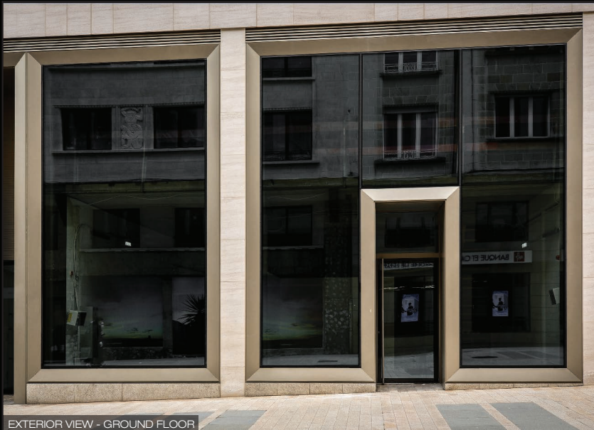
EXTERIOR VIEW - GROUND FLOOR
