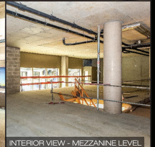
INTERIOR VIEW - MEZZANINE LEVEL
