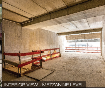
INTERIOR VIEW - MEZZANINE LEVEL
