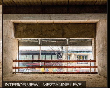
INTERIOR VIEW - MEZZANINE LEVEL
