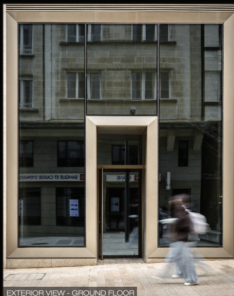
EXTERIOR VIEW - GROUND FLOOR
